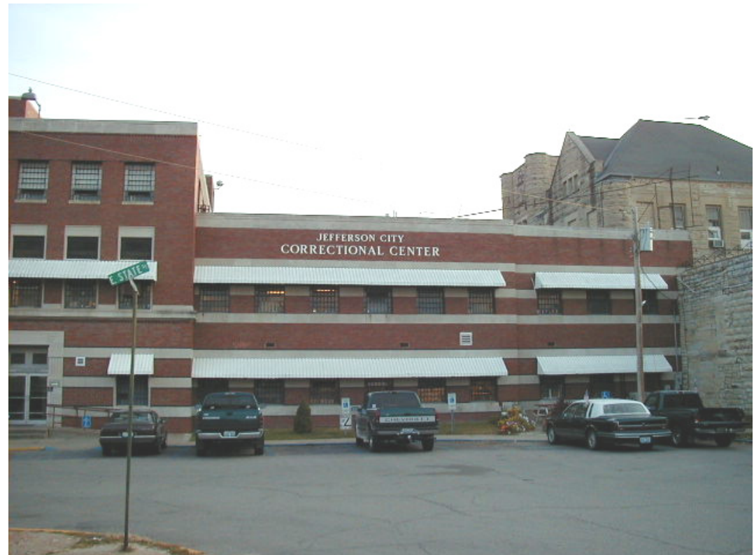
Jefferson City Correctional Facility Administration Building Facing North
